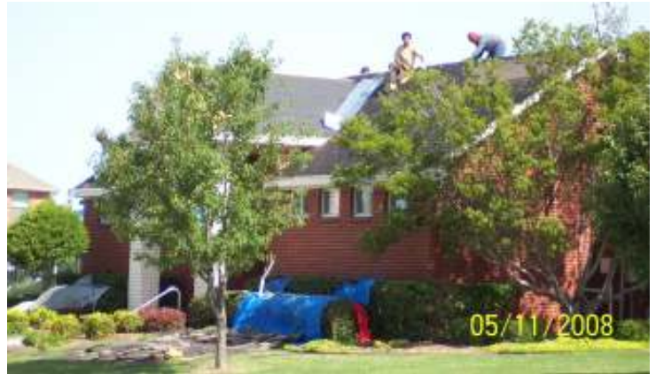
Contractors replacing GPHOA Pool House Roof
